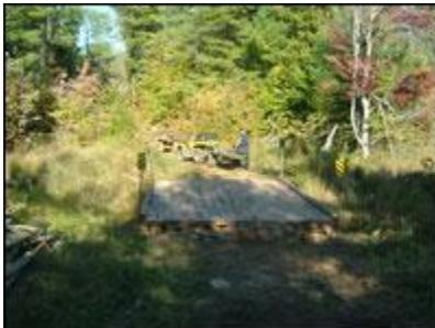
**2004 South Lake Bridge:** 17 volunteers came out to repair the bridge, some from KATVA. Dirt Trax TV was on the scene and shot footage of the club's work for their television show. The MNR had marked 20 trees to be cut down and used for the base of the bridge. They were about 8 inches in diameter and about 20 feet long. Haliburton County Snowmobile Association supplied the decking HATVA supplied the volunteers.
