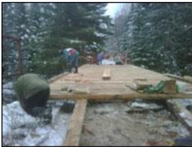
**2010 IB&O Repair:** In late November, five HATVA members removed the decking from a bridge on the IB&O Rail Trail between Gooderham and Irondale. This was a cooperative effort with the Buckhorn Snowmobile Club which completed the job, re-decking it.
